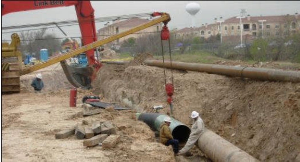
Figure 46. Replacing a piece of pipe. Courtesy Pipeline Knowledge & Development.
