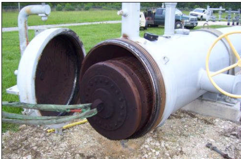
Figure 38. Removing a pig from the receiver. Courtesy Line Star Services Company.
