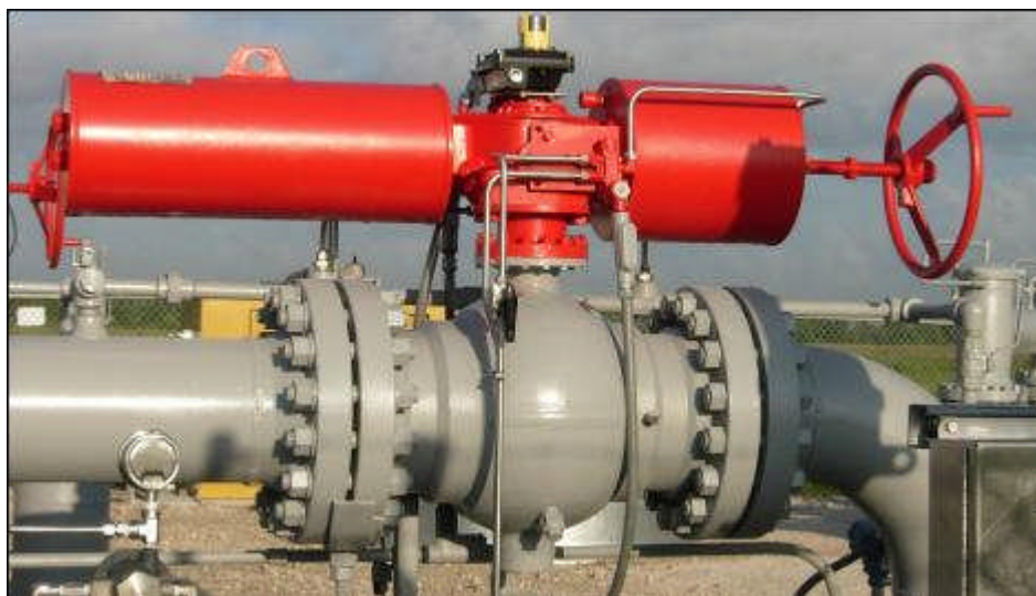
Figure 35. Actuator on a ball valve. Courtesy Pipeline Knowledge & Development.
