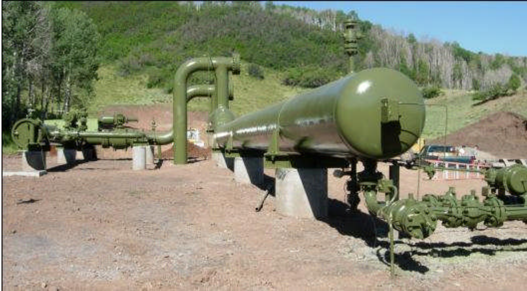
Figure 36. Pipeline slug catcher. Courtesy Pipeline Knowledge & Development.
