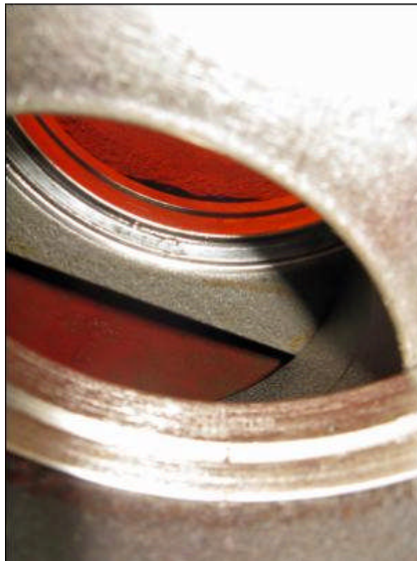
Figure 32. Partially open slab gate valve. Courtesy Pipeline Knowledge & Development.
