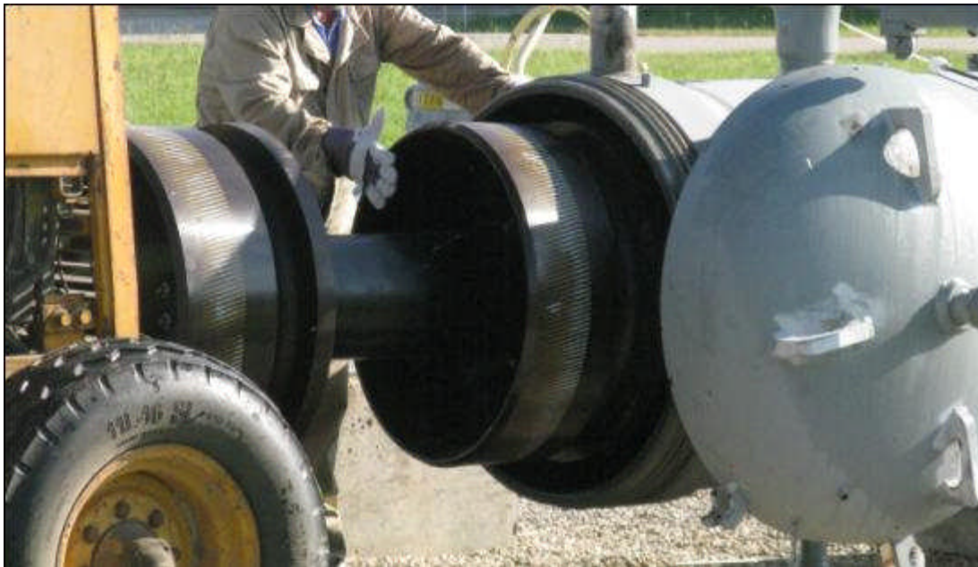
Figure 47. Loading a cleaning pig. Courtesy Pipeline Knowledge and Development.
