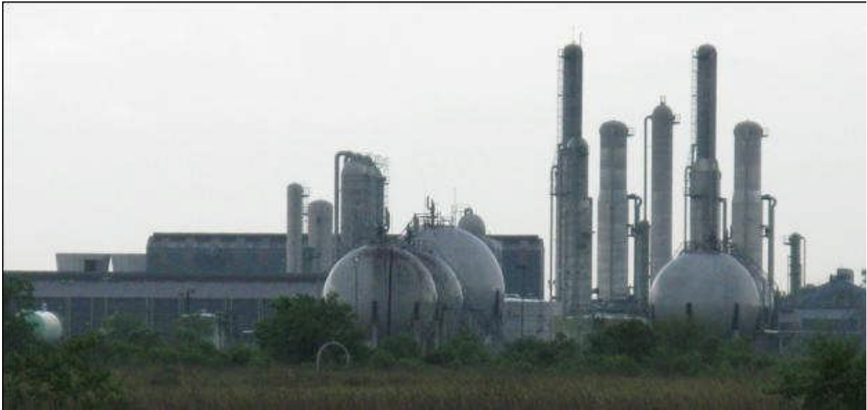
Figure 3. Gas liquids extraction plant. Courtesy Pipeline Knowledge & Development.
