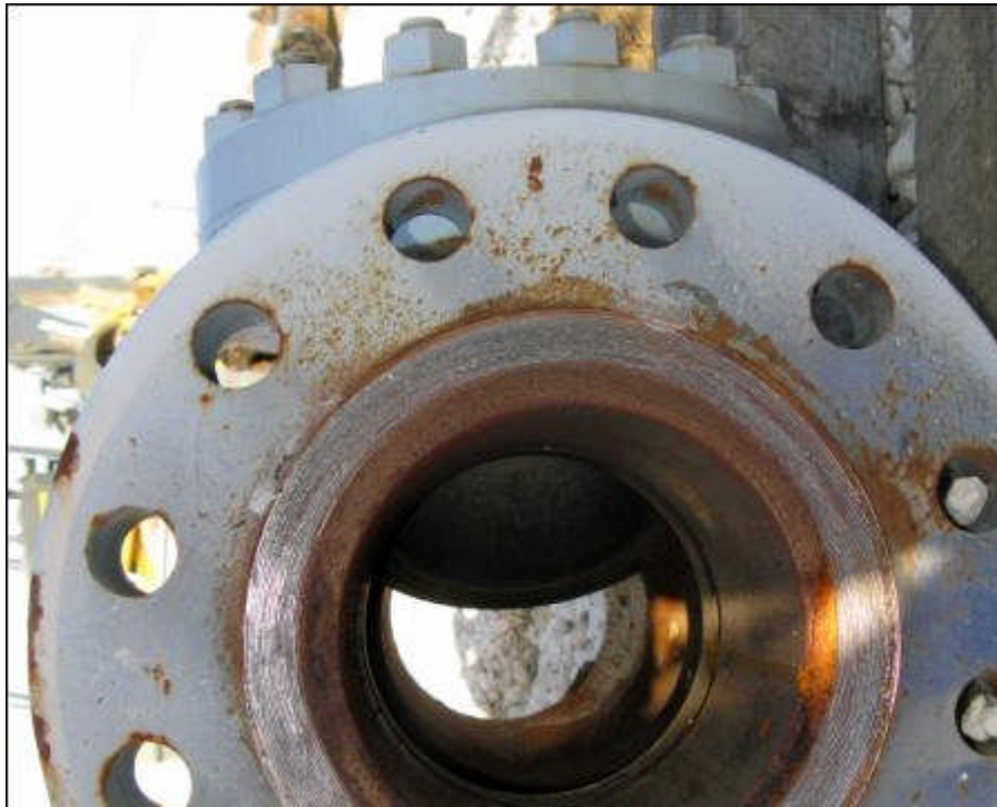
Figure 34. Partially open swing check valve. Courtesy Pipeline Knowledge & Development.
